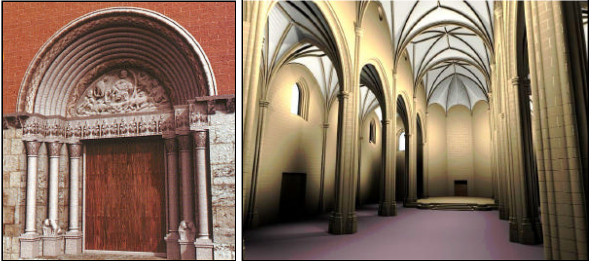
Fig 3. A Romanesque style portico (left) created by means of photogrammetry and a gothic church main nave (right) measured using topography. Photogrammetry is a technique usually used for high detail models with many ornaments while topography is generally used for big structures with less detail.
